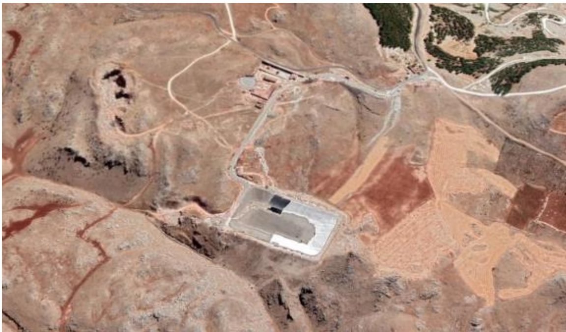
Figure 1. The project site (satellite view)
